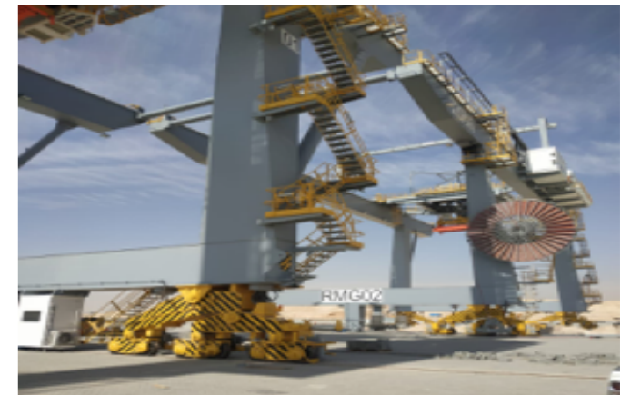
RMG arrived to the yard and settled on the rail
