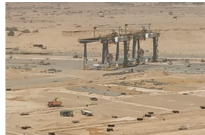
The RTG cranes after erected and ready for commissioning
