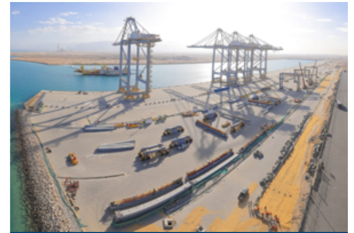
The eight crane have been erected all and they are under commissioning
