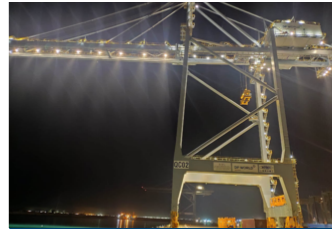
The four crane have been completed the commissioning and now they are under function test
